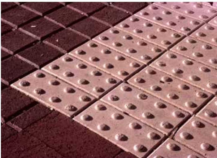
Detectable warnings come in a variety of styles, colors, and materials including brick or concrete unit pavers (left) and steel plates (right).
