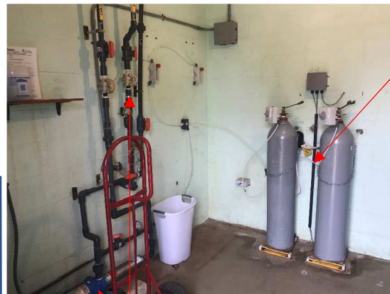
Chlorine Booster Pump & Piping
